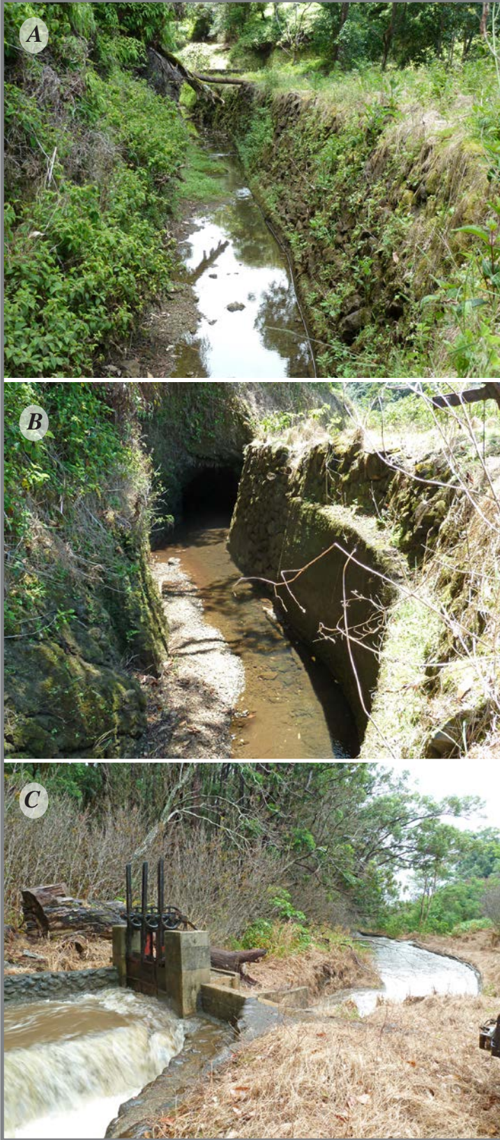
Figure 7. Photographs of three sections of the New Hāmākua and Kauhikoa Ditches, East Maui Irrigation diversion system, east Maui, Hawai'i. A, New Hāmākua Ditch, unlined open-ditch section at 'O'opuola Stream. B, New Hāmākua Ditch, partially lined open-ditch section near Waipi'o Stream. C, Kauhikoa Ditch, lined open-ditch section at 'Ōpana Stream.
