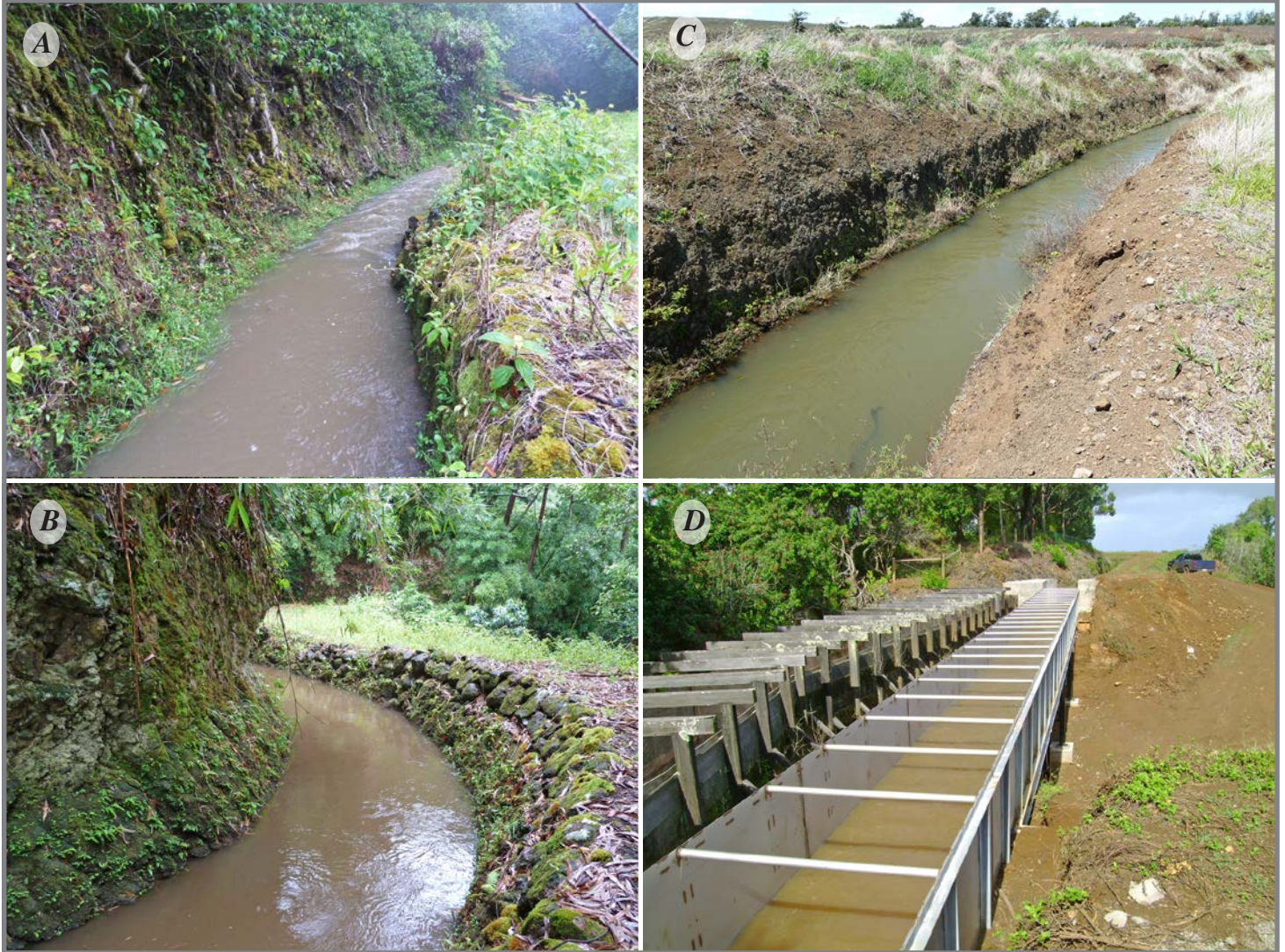
Figure 9. Photographs of Manuel Luis, Center, and Lowrie Ditches, East Maui Irrigation diversion system, east Maui, Hawai'i. A , Manuel Luis Ditch, unlined open-ditch section near Puohokamo Stream. B , Center Ditch, unlined open-ditch section between Kōlea and Punalu'u Streams. C , Lowrie Ditch, unlined open-ditch section near Māliko Gulch. D , Lowrie Ditch, old wood flume and replacement stainless-steel flume near Pe'ahi Reservoir (photograph by Garret Hew, East Maui Irrigation Company).
