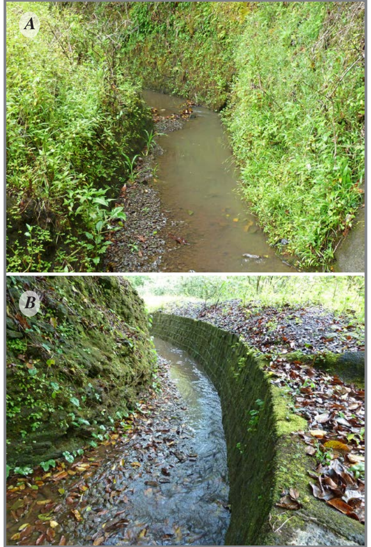
Figure 8. Photographs of two sections of the Spreckels Ditch at Pāpa'a'ea, East Maui Irrigation diversion system, east Maui, Hawai'i. A, Unlined open-ditch section near Ka'aiea Gulch. B, Partially lined open-ditch section near Ka'aiea Gulch diversion intake.
